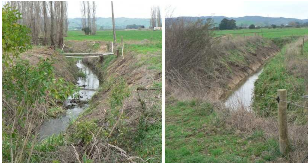
Figure 18: Clearing of farm drains and stream banks can leave soft alluvial soils bare and vulnerable to erosion during storm events (Photo: M. Gibbs; 19 June 2008)
