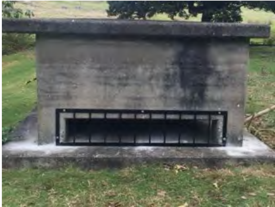
New grates fitted to restrict access into the tunnels
